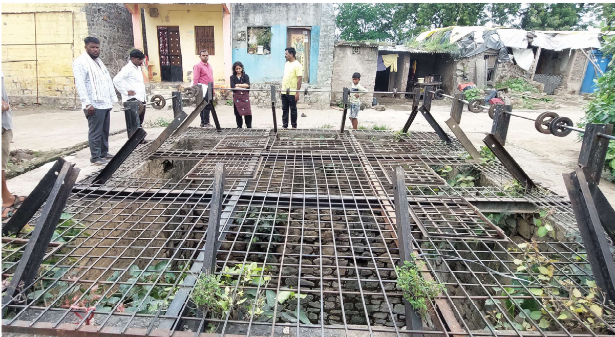
Inspection of water sources
